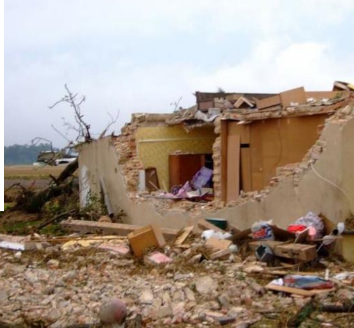
Image 6: F4 damage (strong brick structure, walls partly collapsed) in western Mira close to the Villa Fini, on the other side of the streamer (photo: Alberto Gobbi)
