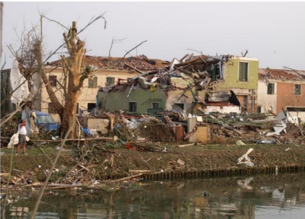
Image 6: F4 damage (strong brick structure, walls partly collapsed) in western Mira close to the Villa Fini, on the other side of the streamer (photo: Alberto Gobbi)
