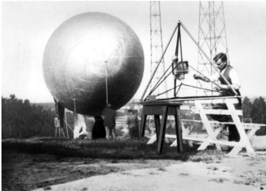
Tethered balloon with a fixed-point-meteorograph at Lindenberg, Germany 1938
